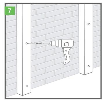
Once drilled, fix the battens to the wall using the expansion screws and wall plugs.
